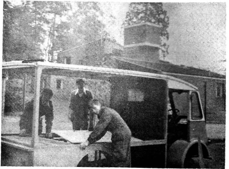
Laying a new floor to the milk float A/Ptes McDonald, Cherry and McGaughey
